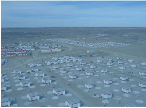
Completed construction project of main camp expansion ahead of schedule at Oyu Tolgoi project
