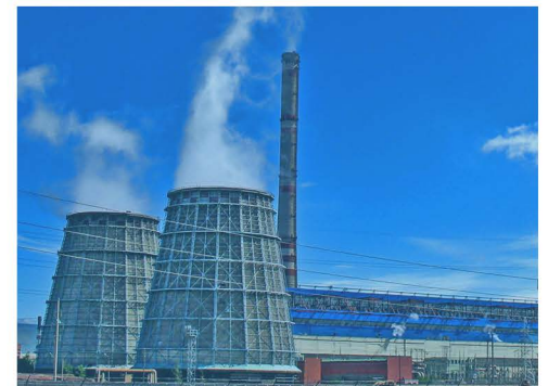
Established to provide services to thermal power plants in UB.
